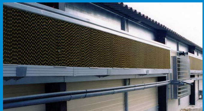
MODULOS INTEGRALES (con bomba, tuberías y regulación exterior) INTEGRATED MODULES (with pump, pipes and external regulation)
